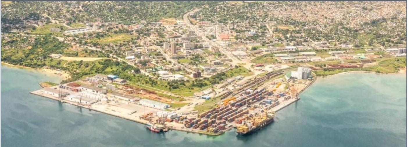
Figure 24: Port of Nacala, Mozambique
