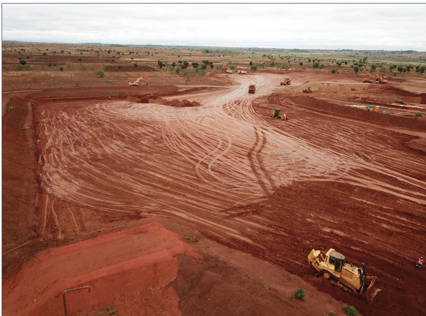
Figure 18: Backfilling of test pit during the Pilot Phase
