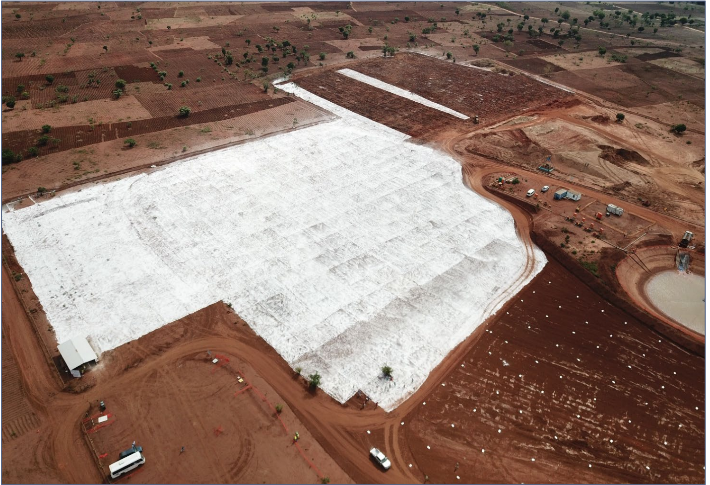
Figure 29: Introduction of lime at the backfilled test pit
