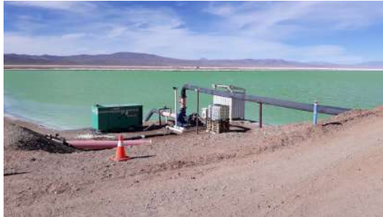
Figure 14.6 Evaporation Ponds – Transfer Pump Station
