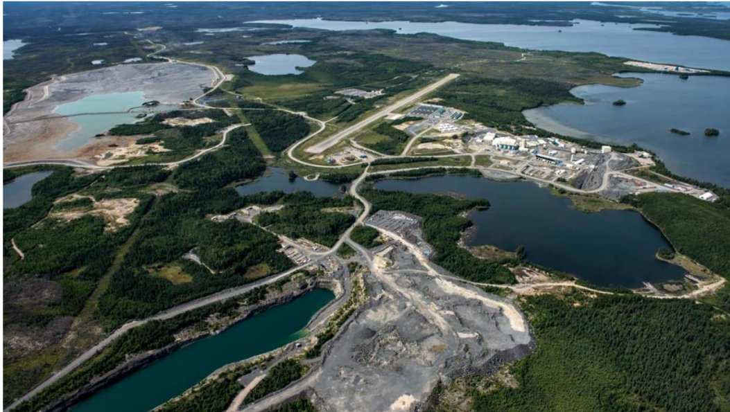
Figure 18.2 – Aerial View of the Project
