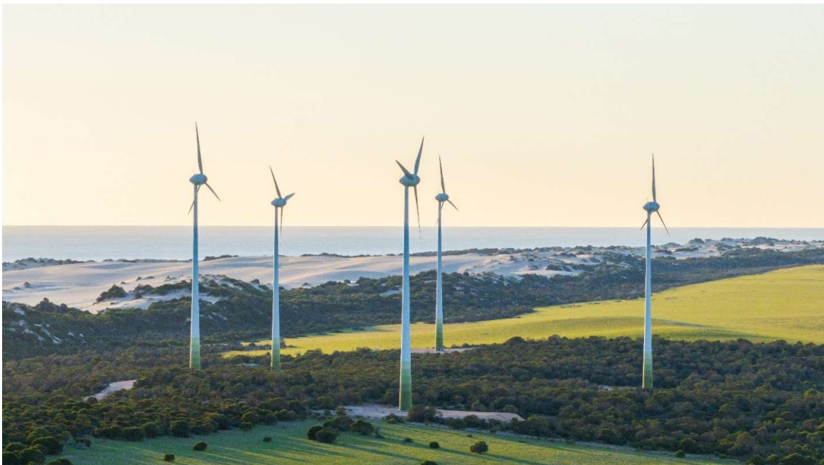
Figure 6 Lucky Bay Wind Farm
