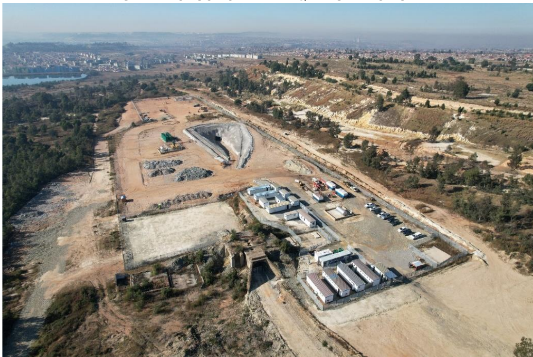
IMAGE 4: PRODUCTION READY QALA SHALLOWS MINE
