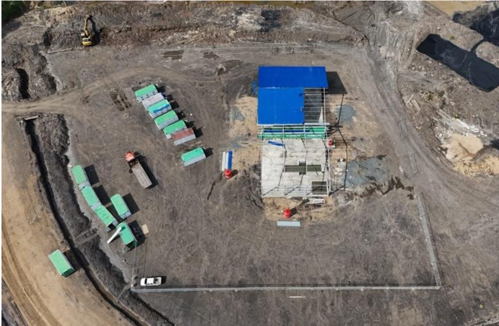
Magazine Warehouse Construction Progress Pit 3 (Aerial View)
