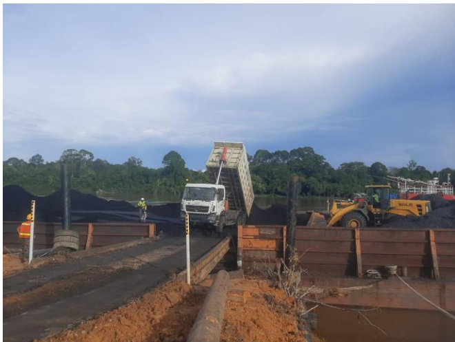
Barge Loading (Batu Tuhup Jetty)
