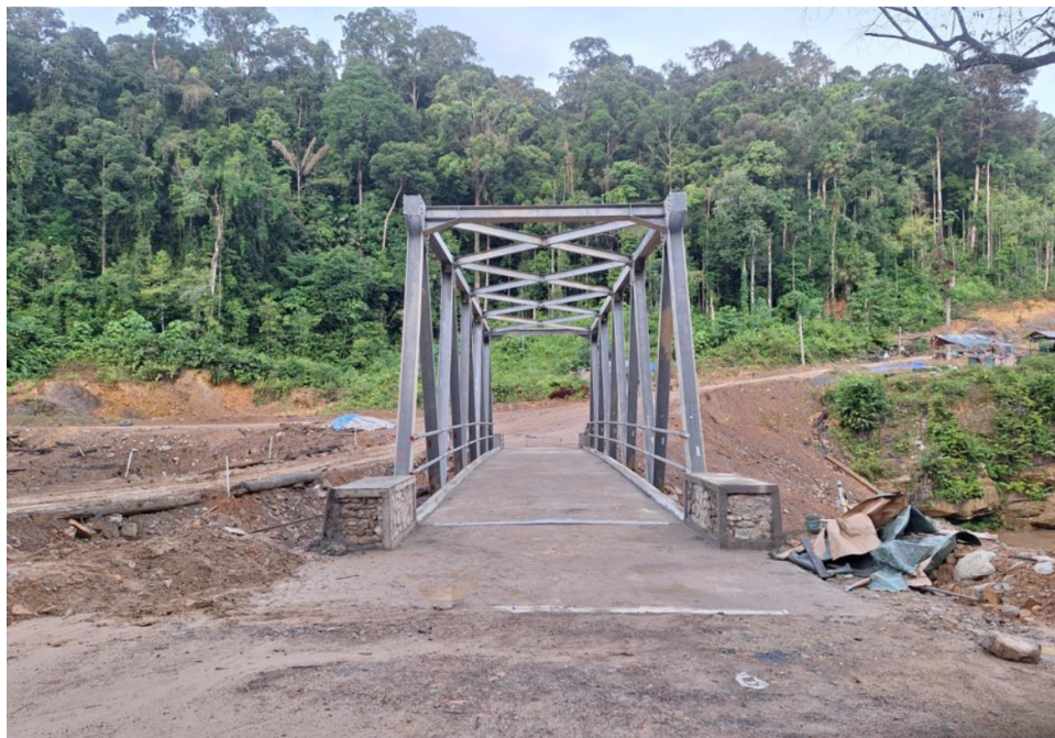
Mohing Bridge KM70
