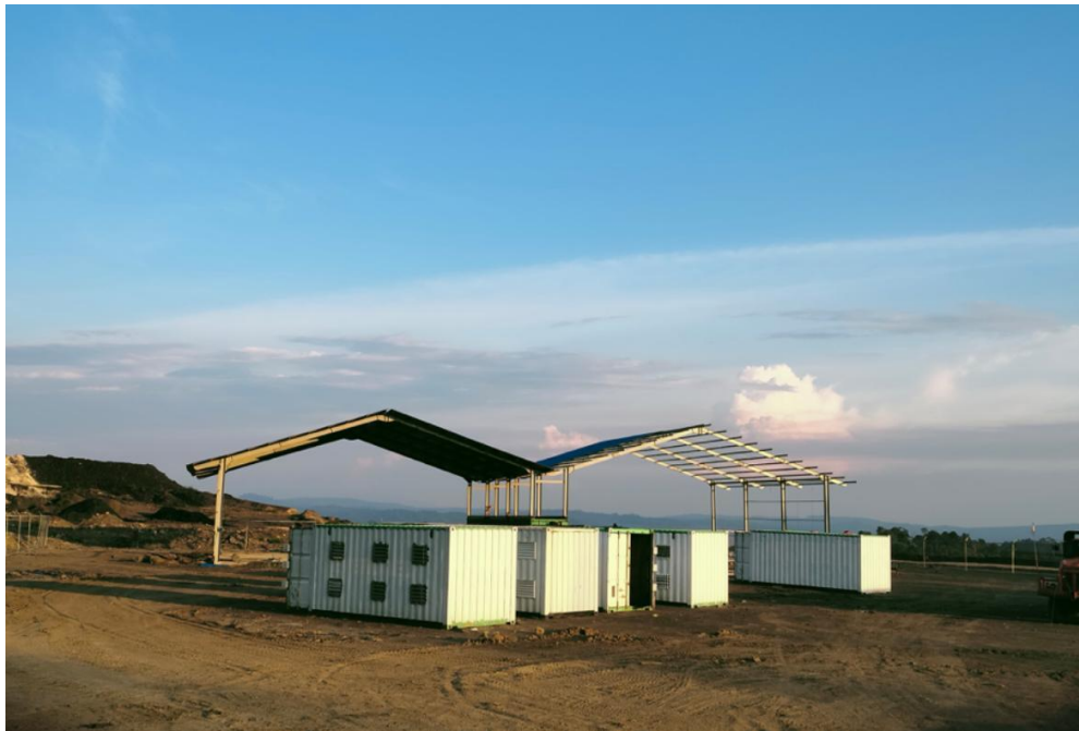
Magazine Warehouse Construction Progress Pit 3
