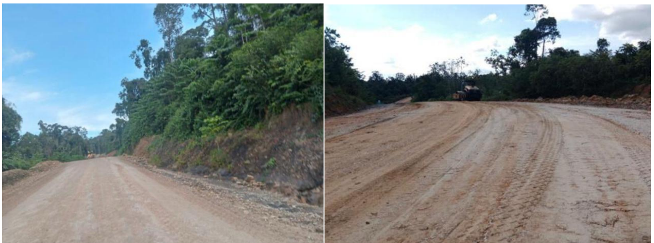
Road Maintenance Works
