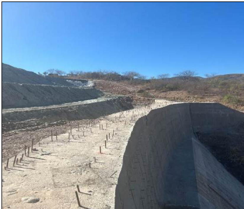
FIGURE 14.14 NEWLY CONSTRUCTED TAILINGS BERM FACILITY
