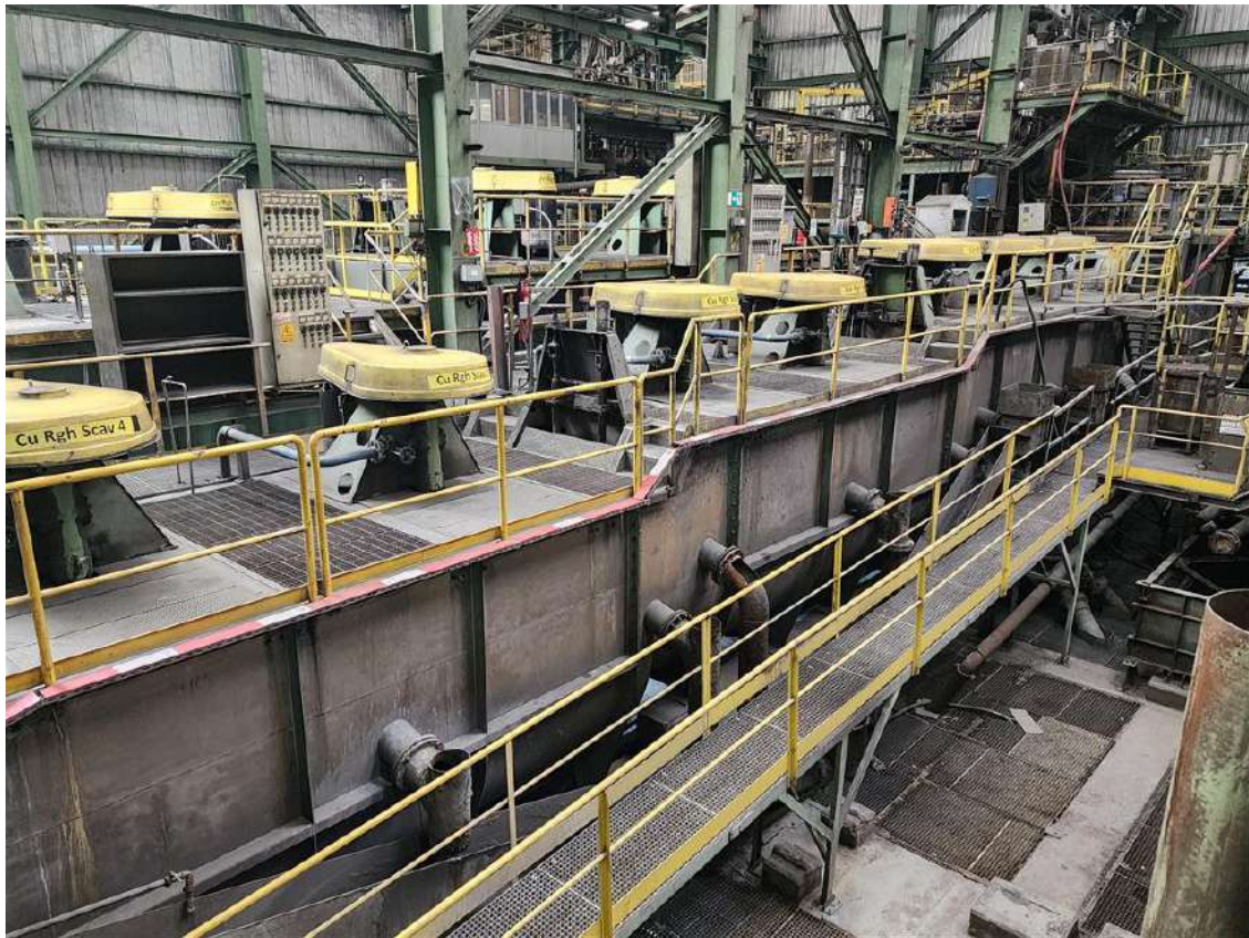
Figure 17.8 Cu Rougher scavenger cells in good condition
