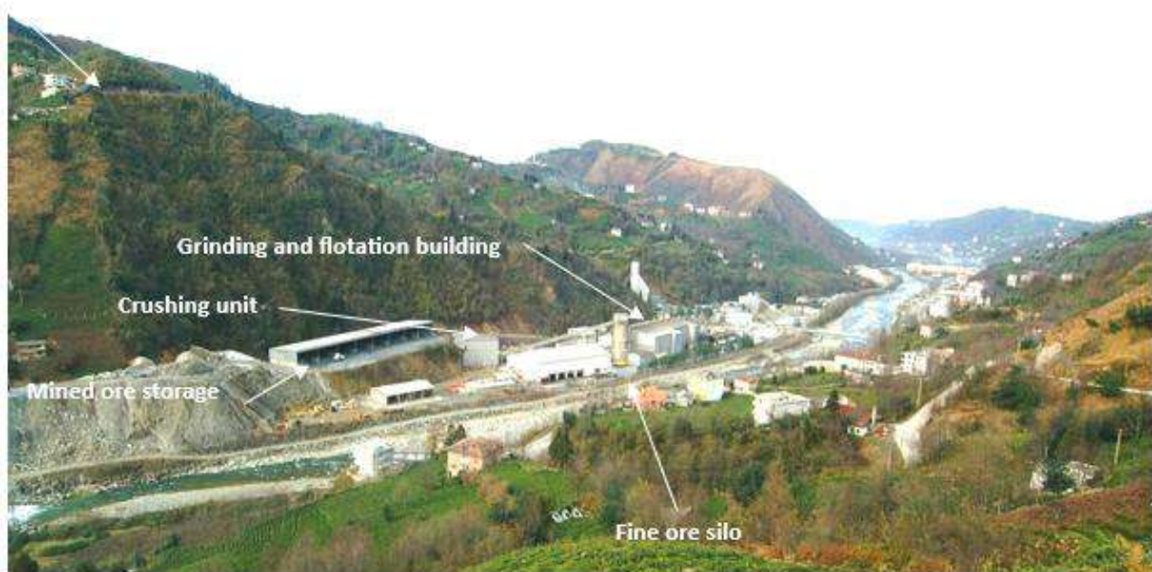
Figure 17.3 Çayeli Operations surface installations
