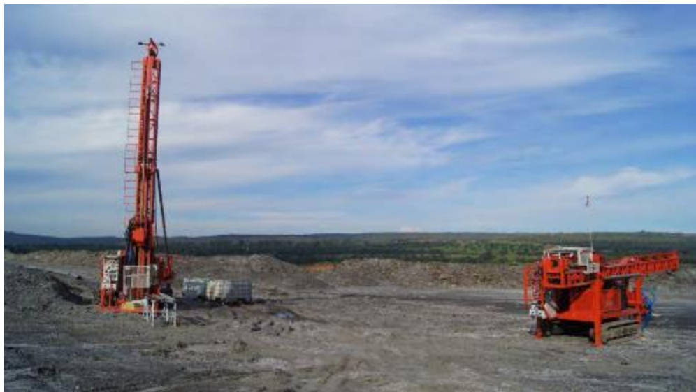
Figure 10-1: Drill rig operated by KBM team in pit area
