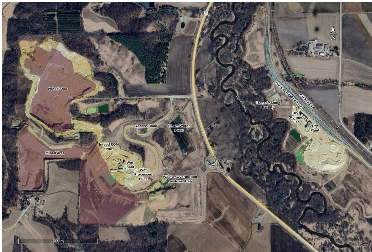
Figure 16.1: Overview of the Blair Facility Showing Significant Infrastructure. The illustration includes the location of the active mining area, wet and dry plant facilities, product storage areas, waste storage areas, haul roads, rail loading terminal, rail car holding yard and proposed direction of future surface mining.
