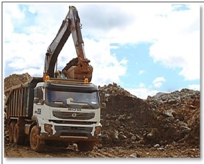
Photo 11. Ore retrieving and transferring operation.
