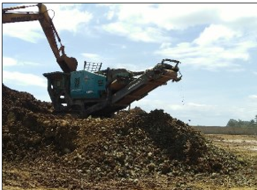
Photo 15. Mechanical crushing using mobile crusher (MC)
