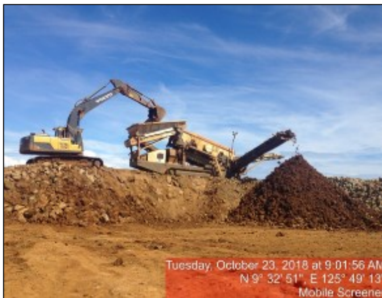
Photo 12. Mechanical screening using mobile screener
