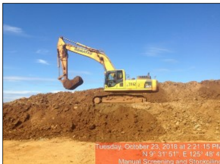
Photo 13. Sizing and sorting using track excavator (TX)
