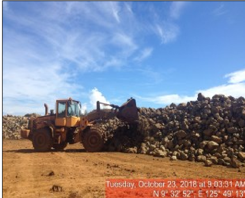
Photo 14. Scraping and stockpiling using wheel loader (WL)
